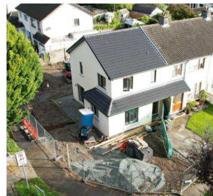
Infill site - 169A Clonsilla Road
